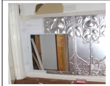
Marked out panel cut out for A/C vent
