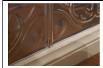
Show's nail holding in place temporarily prior to permanent fixing.
