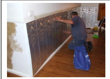
Showing marking out prior to installing
