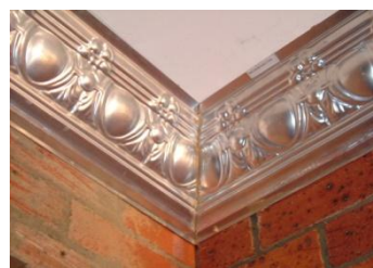
8/Shows example of finished Mitred cornice.
