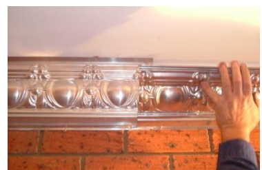
9/Shows putting cornice in the mounting strips overlapping each cornice.
