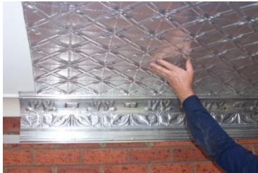
1/Shows the Cornice Mounting Strip which is To be installed first. This can be install with a Small nail, tack or screw. Lip is to face out.
