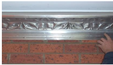
2/ Shows the cornice slipping into the Mounting strip straight over an existing Gyprock Cornice. There is no need to remove old Cornices unless The old is larger than the new.
