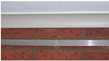
1/Shows the Cornice Mounting Strip which is To be installed first. This can be install with a Small nail, tack or screw. Lip is to face out.
